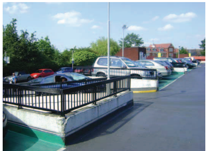
Tesco multi-storey car park
