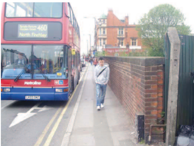
The bridge over the railway lines
